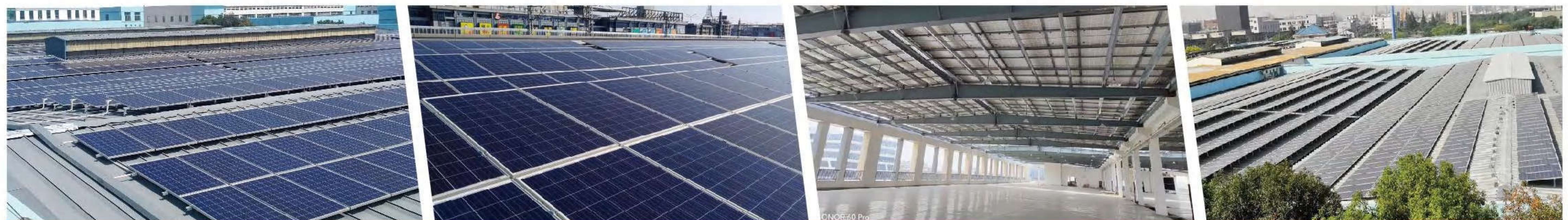
▶ The BAOJIANG Industrial Zone Project in Shaoxing
