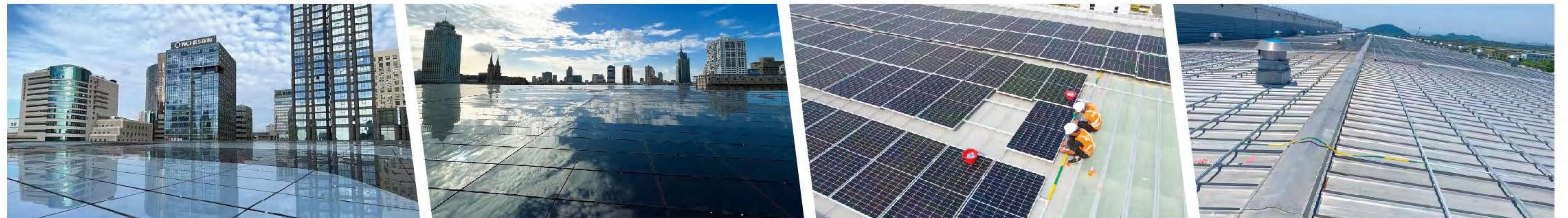
▶ Tianyi Plaza Green Low Carbon Parking Building
