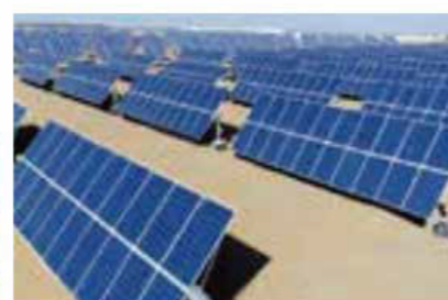
OFF-GRID PV station
