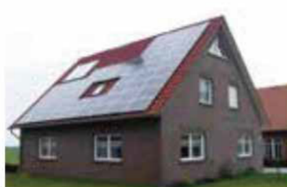
Home Photovoltaic System
